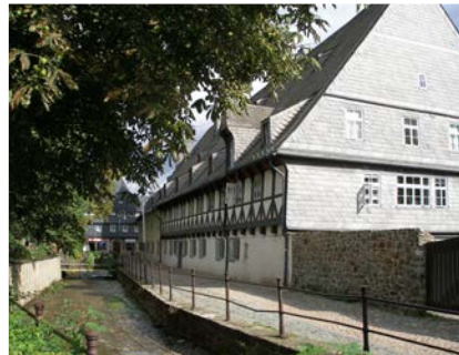
Almshouse "Great Holy Cross" Stone chamber: 12th c. Hall: 1256 Extended: 1537
