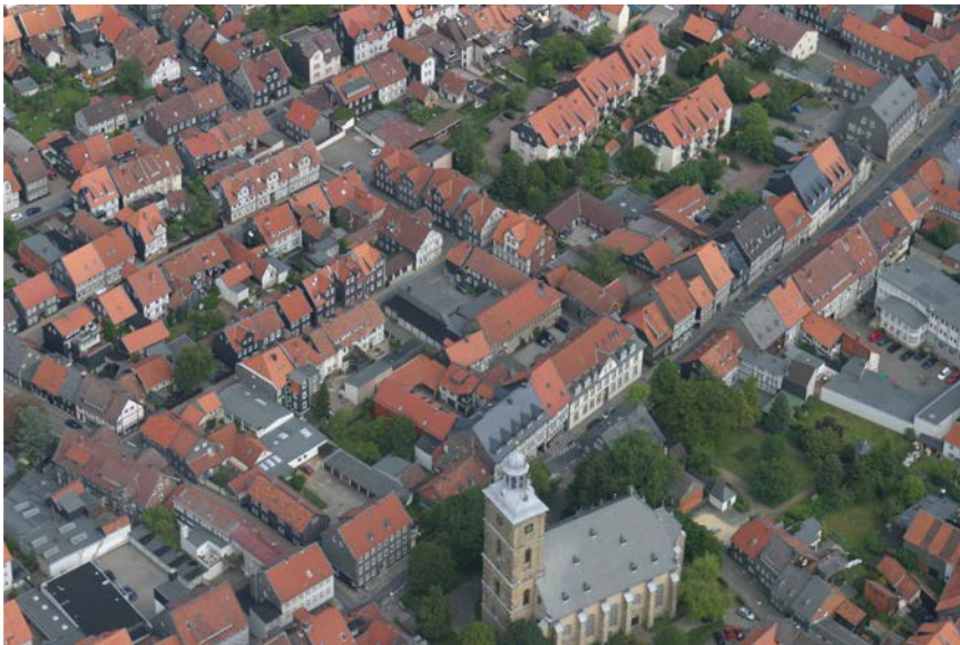
View of a part of the lower town with development within the blocks
