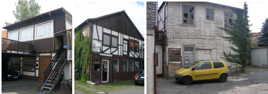
Examples of formerly used buildings in the lower town (without value as historic monuments)
